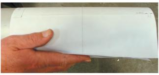
1. Wrap paper template around roller tube, the end you want to install the Daisy Power motor and controls
