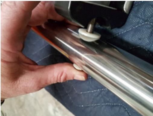
3- Fit one end of a ladder tread over the M8 x 60 ensuring the large nylon washer is in between the rail & the tread end
