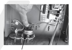
pressure switch adjustment screw
